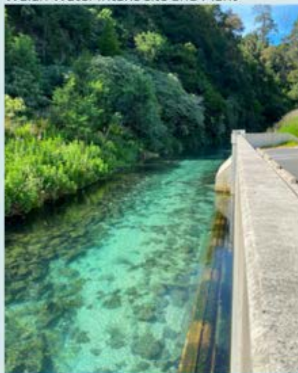
Waiari Water Intake site and Plant
